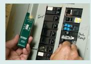
The receiver indicator unit will indicate voltage present. When the user opens the splice or breaker, the voltage present indication stops, thereby identifying the AC wire.
