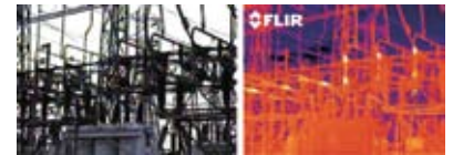
Substation - A wide view of a substation can quickly show areas where unwanted high resistance connections exist. Electrical current passing through a resistive connection produces heat; electrical systems get hot when connections loosen or corrode and power is not properly transmitted — no other predictive maintenance technology is as effective for electrical inspections as IR thermography.
