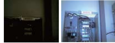
Graphs 4.7 Below visual images taken in a poor lighting environment (i.e. electrical cabinet) however the second image was taken by a camera with visual target illuminator/ lamp.
