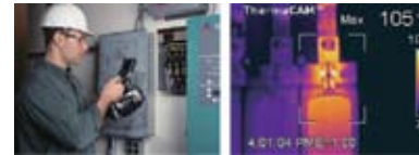
Electrical - Infrared testing is used as a means to detect potential circuit overload or areas of unusually high electrical resistance, allowing electricians to replace the circuit before failure, eliminating costly downtime or further damage to the electrical system.
