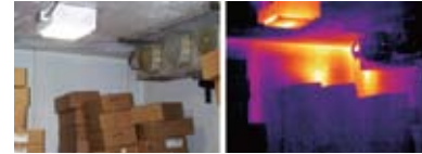
Freezer - Poor insulation in a walk-in cooler
