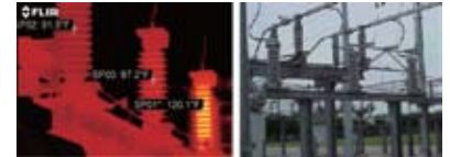
Regular IR Scans Keep the Lights On - Electric companies must have reliable power lines to provide their customers with the service they expect and deserve. Unfortunately, when lightning arresters fail, the whole system hangs in the balance. Regular inspections can help prevent power outages by detecting bad lightning arresters in substations and faults in distribution lines.
