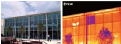
Building diagnostics - Infrared testing is used to detect heating & cooling loss or moisture problems due to insulation deficiencies or construction issues.
